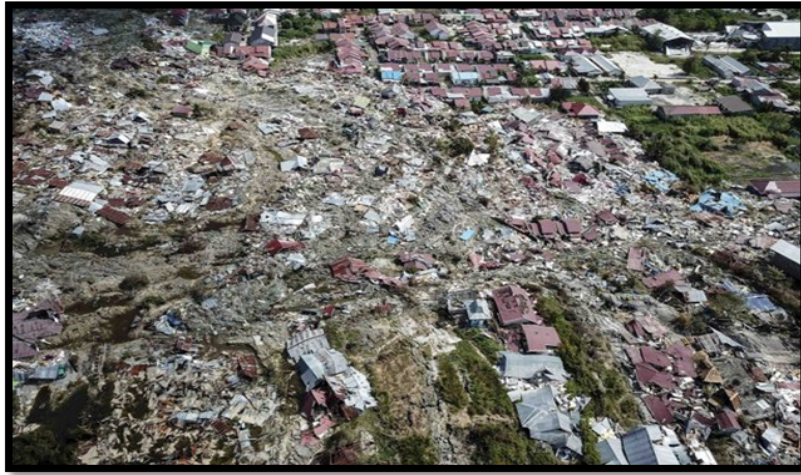
Figure 1. Damage due to the Palu earthquake in the Petobo Region 5
