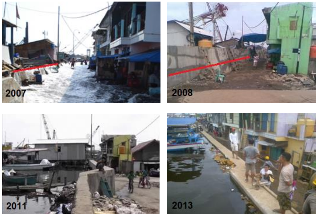
Figure 10. Illustration of dyke “sinking” in Pluit area north of Jakarta. In 2007, around 1 meter of dyke failed to protect the land, while 2008 another 1-meter elevated dyke would soon after 2013 would probably fail again
