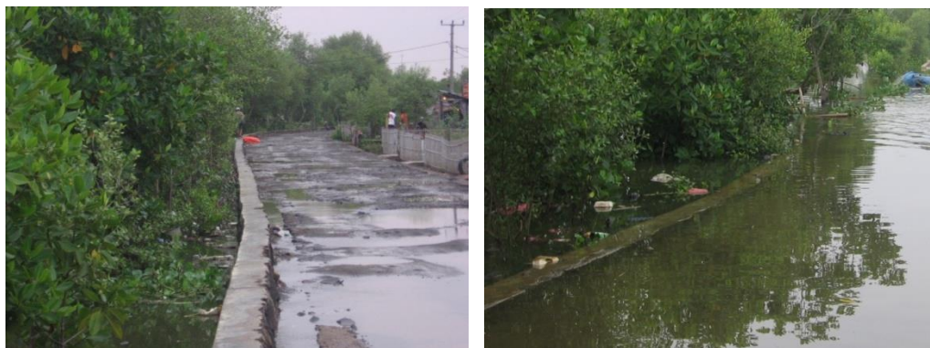
Figure 13. Mangrove and dyke that supposed to protect the land from tidal inundation in Pondok Bali Blanakan area, nevertheless through times the area has suffering again tidal inundation
