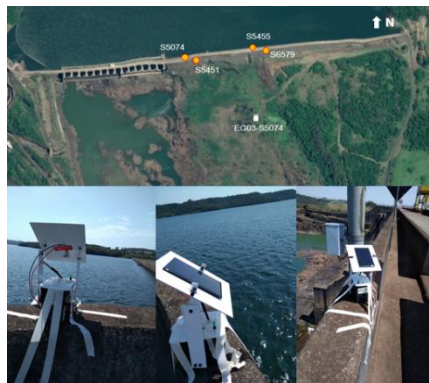
Figure 17. Sensors distribution in the dam for the second test
