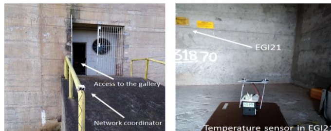
Figure 15. EGI21 temperature sensor installation
