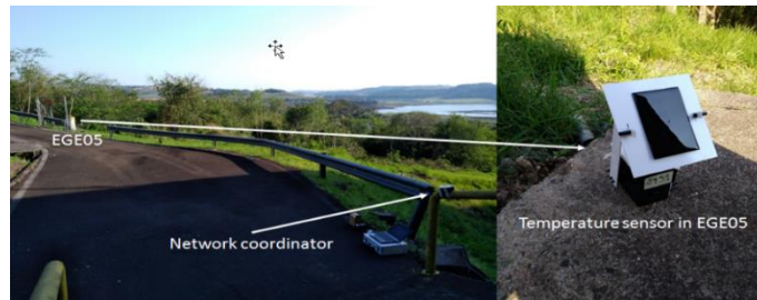
Figure 13. EGE05 temperature sensor installation
