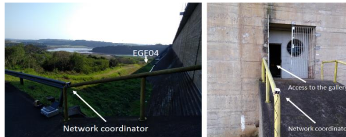
Figure 14. EGE04 temperature sensor installation
