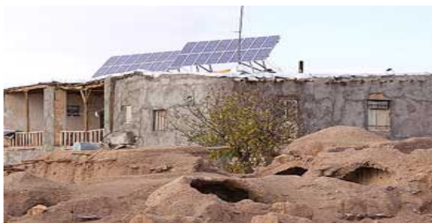
Fig. 6 Solar power in 2 villages of Koohrang in Chaharmahal and Bakhtiari province.
