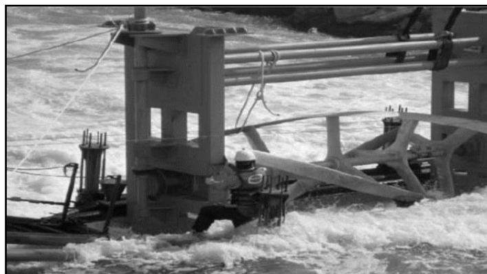
Fig 1. Gorlov Helical Turbines being installed in South Korea (Chakka, 2015)
