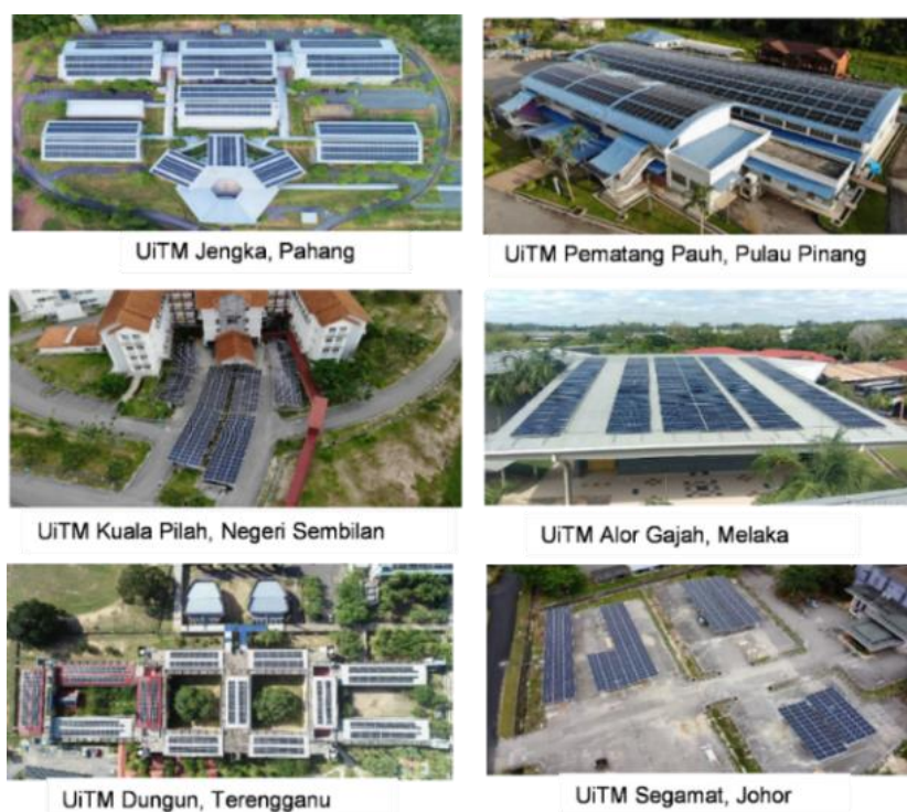
Fig. 1 UiTM campuses with solar PV rooftop under NEM 2.0
