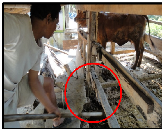
Figure 2. A user shoving the cow-dung into the inlet and then adding it with water to make it more aqueous. (Source: author)
