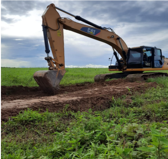
Figure 2. Land clearing by excavator
