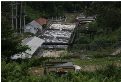
Gambar 3. Kolam Pengolahan Air Lindi TPA Regional Piyungan
