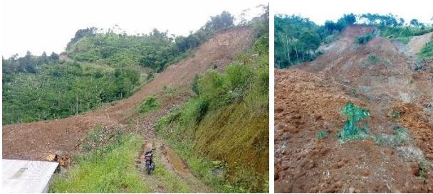
Figure 9. Landslide Condition in Sarwodadi, Pejawaran, Banjarnegara
