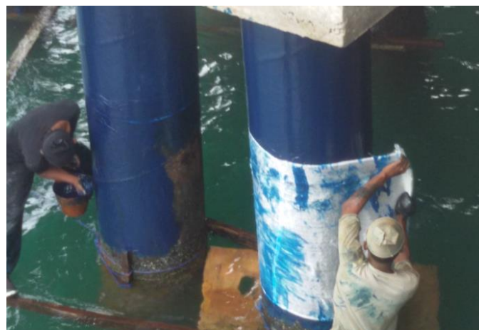
Figure 15. Composite Wrapping Installation
