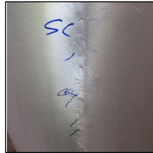
Figure 6. Former Stopper Defect
