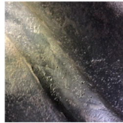
Figure 7. Arc Strike Defect
