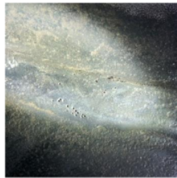
Figure 5. Surface Porosity Defect
