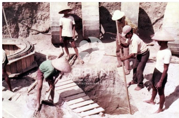
Figure 1. Digitized archival photograph showing manual excavation during the foundation-laying phase of the Kartini Nuclear Reactor construction (source: National Archival Information Network – JIKN, https://jkn.anri.go.id/deskripsi-arsip/1-penggalian-tanah-peletakan-pondasi-paku-bumi-dilakukan-pekerja-secara-manual )
