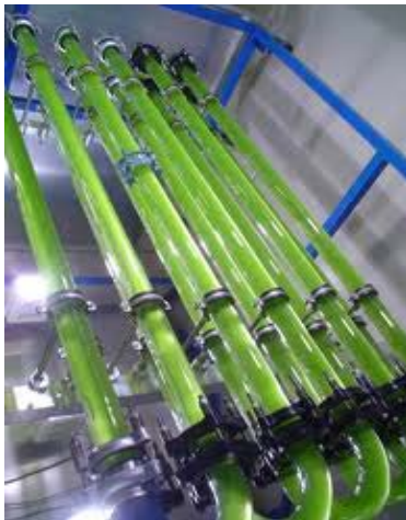
Gambar 4. Instalasi tubular photobioreactor
