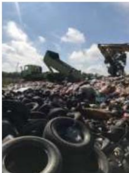
Figure 1. Landfill treatment process with Excavator
