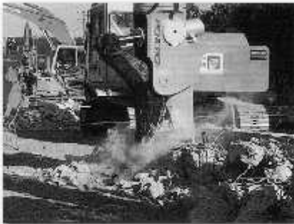
Figure 2. Blasting of Concrete Structures (Kasai, 1986)
