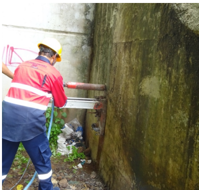
Gambar 2. Pengambilan sampel core drill beton
