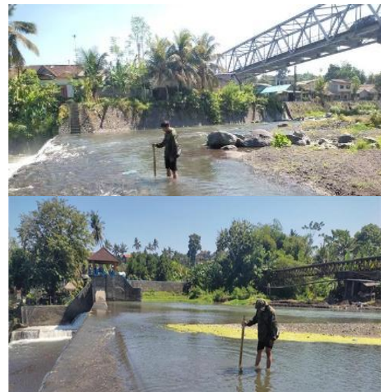
Figure 3. The check dam sedimentation
