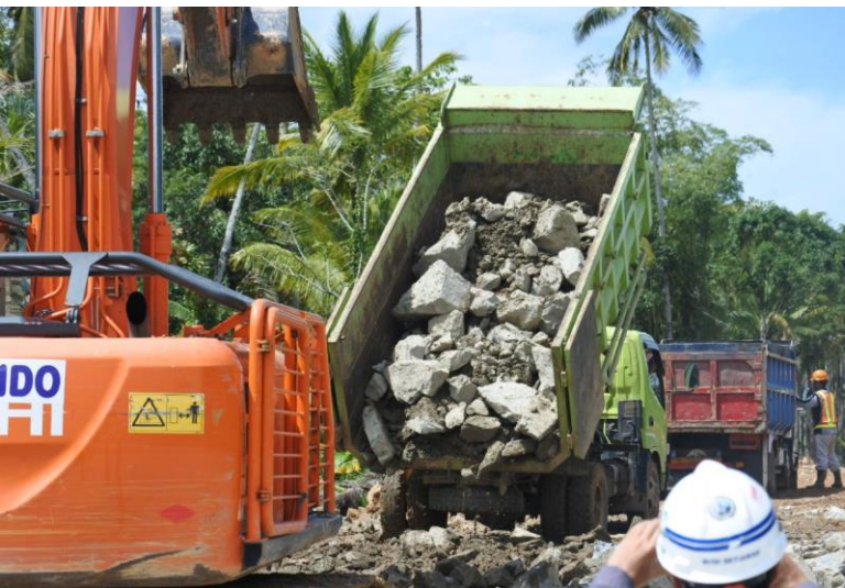
Embankment work using Boulder Stone to accelerate the progress
