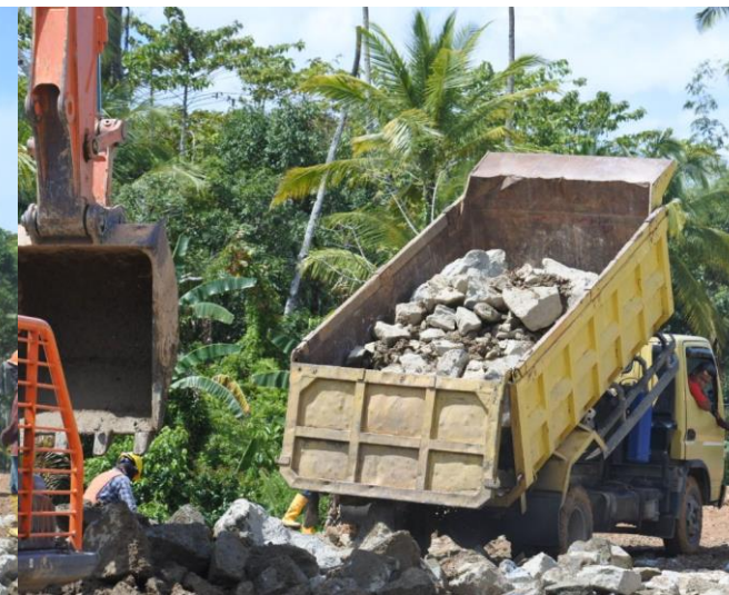
Embankment work using Boulder Stone to accelerate the progress
