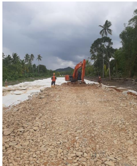
Embankment work using Boulder Stone to accelerate the progress
