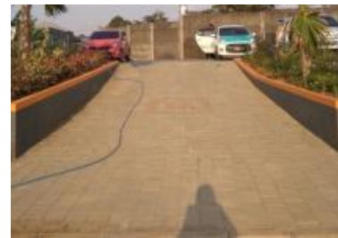
Gambar 5. Kondisi Ramp (Christy, 2018)
