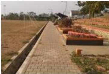
Gambar 2. Kondisi Jalur Pedestrian (Christy, 2018)
