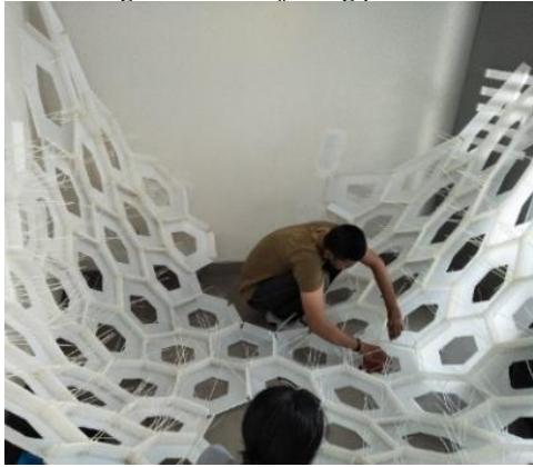
Figure 13. The result of joining the panels to form a shell
