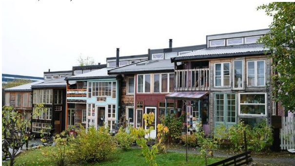
Figure 2. The five self-built houses in Svartlamon, source: http://www.eksperimentboliger.no/
