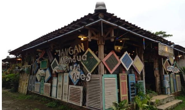
Figure 11. Application of waste to wall elements (Google maps accessed on 12 December 2024)
