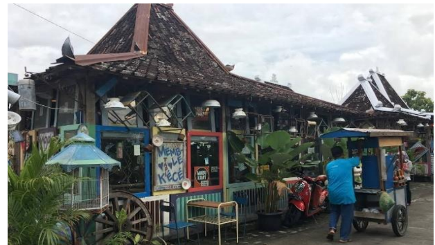
Figure 9. 80's Café Leaks in Bantul (Google maps accessed on 12 December 2024)
