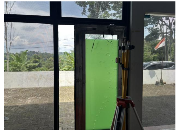
Fig 3. Installation view of the photobioreactor façade system, representing the baseline niche innovation in this study.
