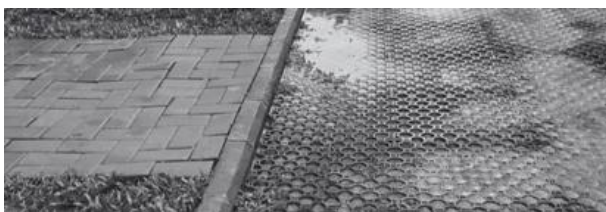
Figure 7. Transition surface rubber and paving blocks on the path to the ramp Ali Sadikin building. (Author, 2025)
