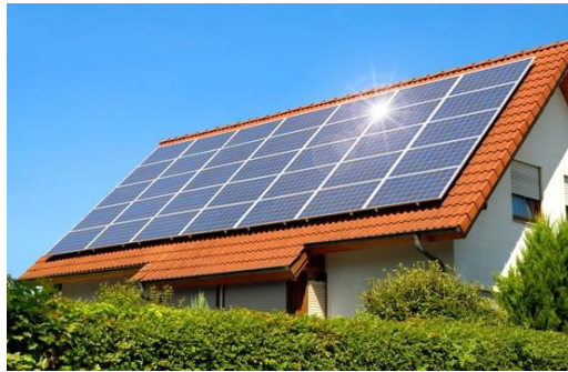
Figure 2. Solar panel roof (Puiu, 2022)
