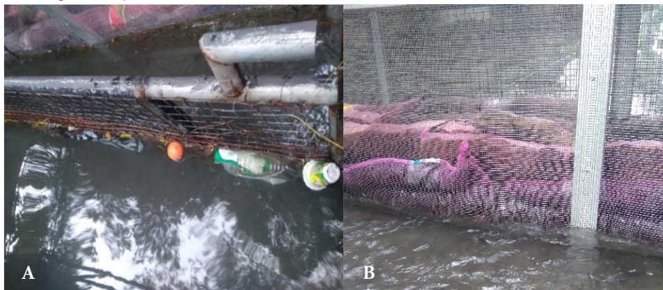
Figure 4. Installation of SPA filter media: (a) rear view; (b) front view
