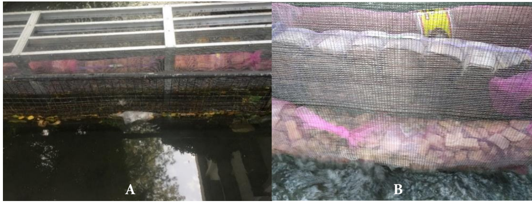
Figure 2. Installation of SPZ filter media: (a) rear view; (b) front view
