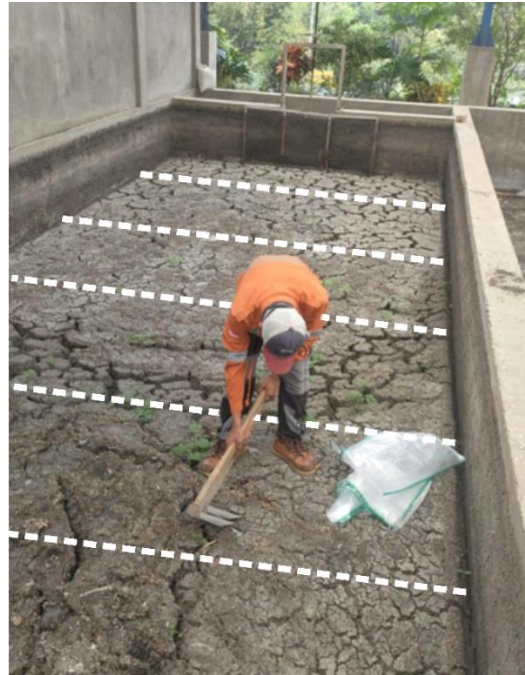
Figure 1. Sampling of fecal sludge in the sludge drying bed
