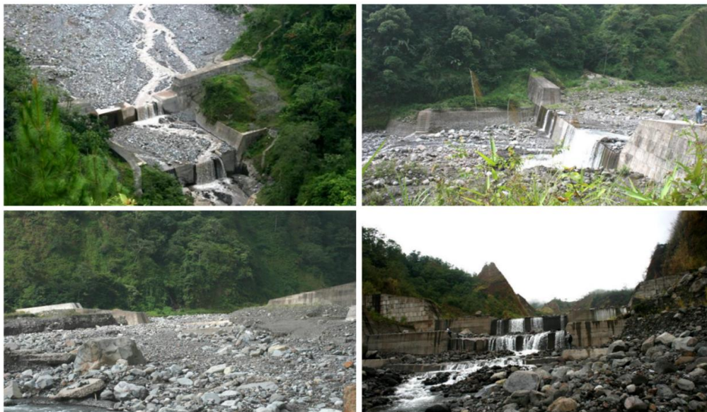
Figure 10. Condition of existing sabo dams in the Bili-Bili Reservoir catchment area Source: BBWS Pompengan Jeneberang (2017)
