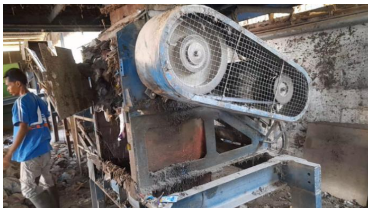
Figure 2. Crusher operated by local community to process dry mixed waste for refuse-derived fuel (RDF) production
