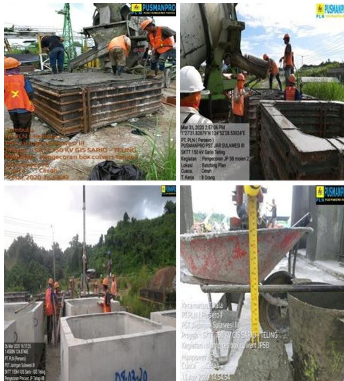
Gambar 6. Pengecoran Beton Box Culvert Joint Pit (Sumber: PLN)
