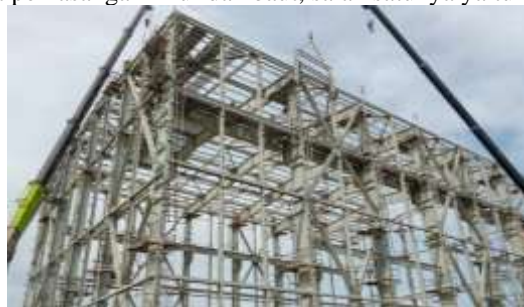
Gambar 2. Steam turbine building
