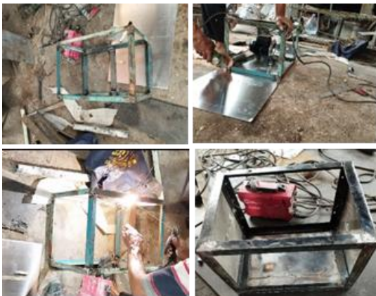
Figure 6. Steel Frame Manufacturing Process Gambar 6. Proses Pembuatan Rangka Besi
