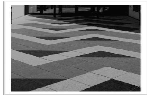
Figure 2. Colored Paving Blocks
