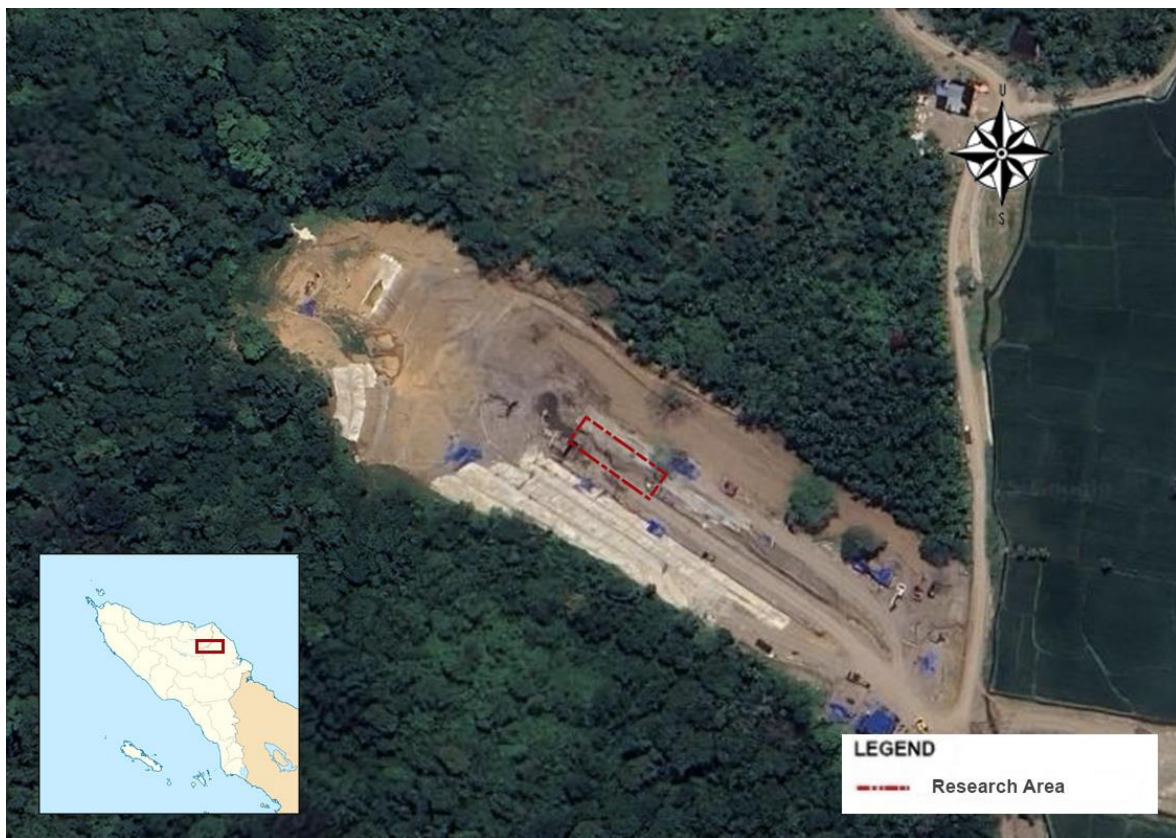
Figure 1. Landslide Location at the Inlet of the Rukoh Directional Structure, Aceh Province.
