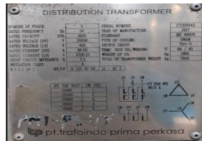
Gambar 2. Name Plate Transformator 3 MVA
